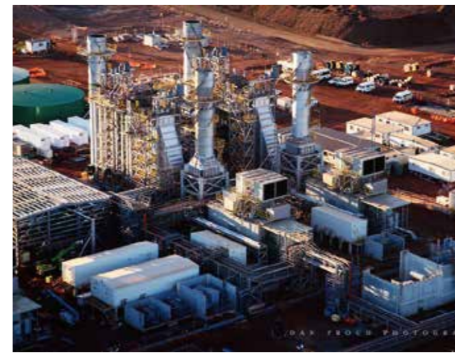
Sino Power Station
