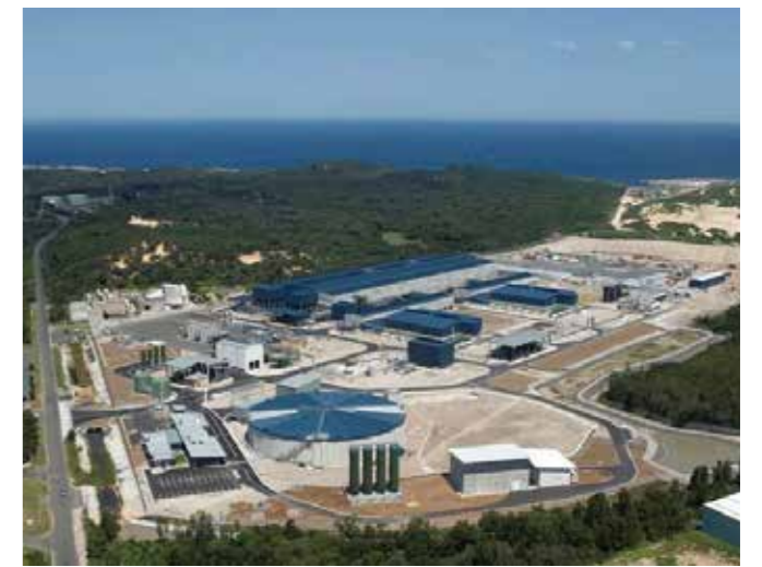
Sydney De-Salination Plant, New South Wales
